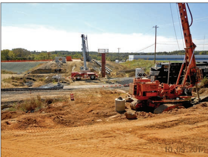
P-5208 Haydock to Junker - Caldwell Road bridge
