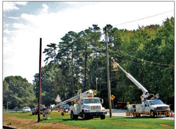
P-5206 Reid to N. Kannapolis - Landis Utility Work
