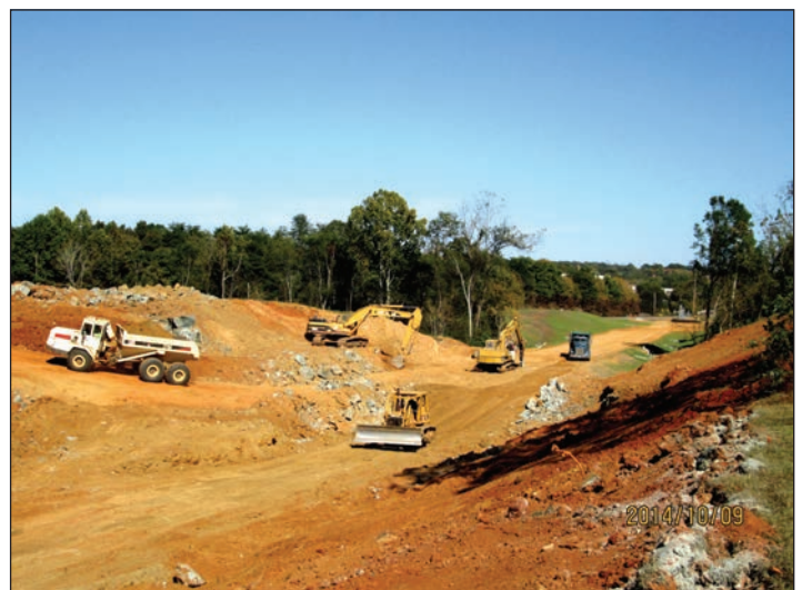
P-5205 Graham to Haw River Grading
