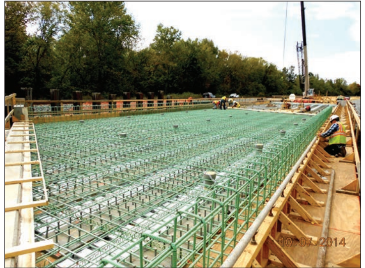
C-4901 Bowers to Lake - Bridge over Hamby Creek
