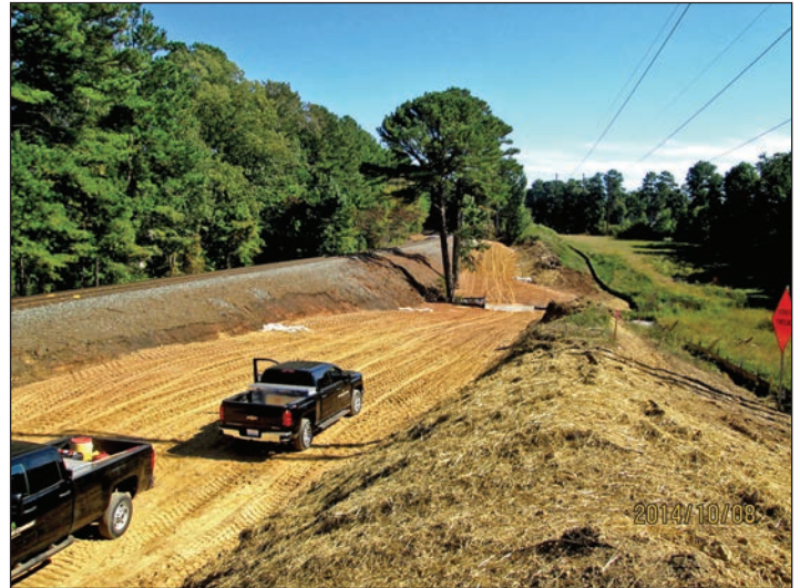
P-5201 Morrisville Parkway, west approach to bridge
