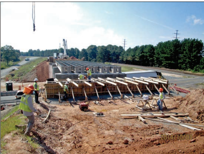
U-4716 Hopson Road bridge construction
