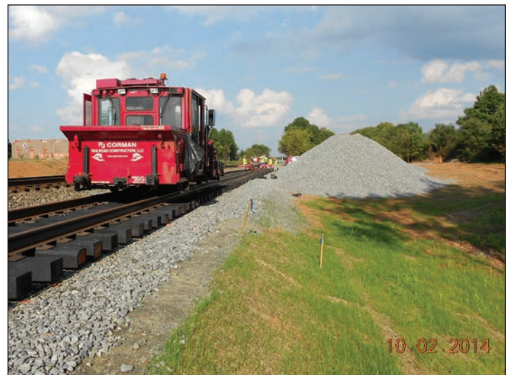
P-5208 Haydock to Junker - Track Construction
