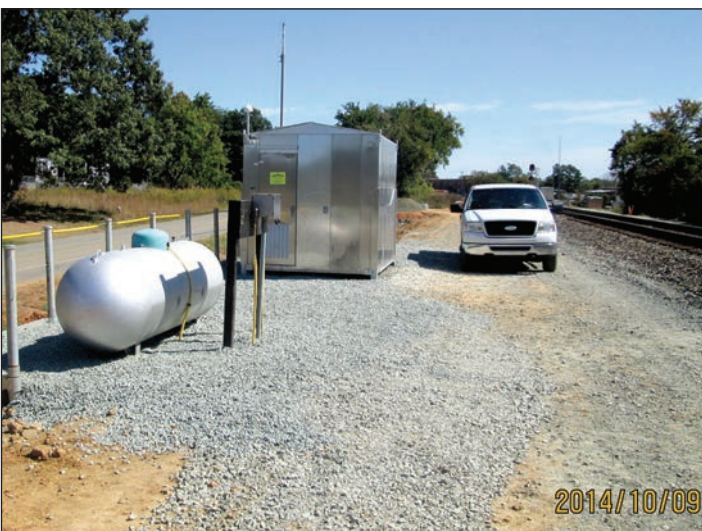
P-5205 Graham to Haw River, signal installation
