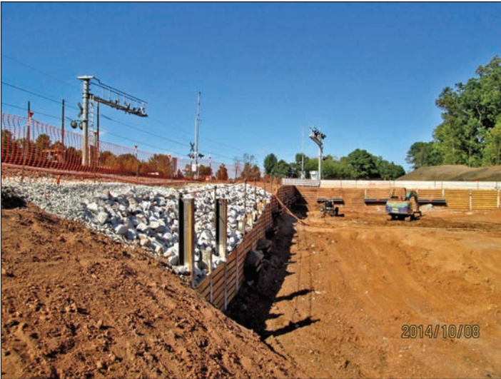
P-5201 Morrisville Parkway grading
